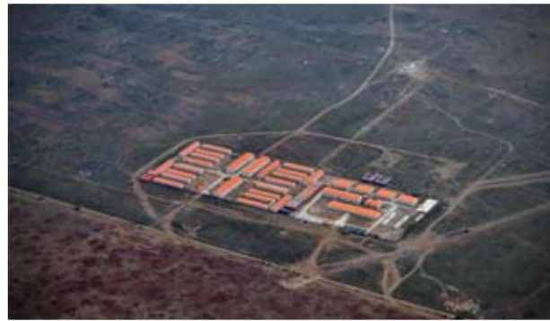
AGANANG CONSTRUCTION CAMP SITE
